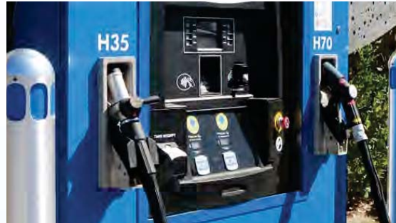
This hydrogen fuel station offers a half-pressure fill, equivalent of a conventional half-tank, and a full fill.
