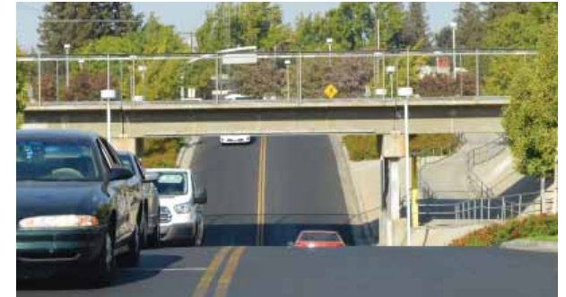
The FCC under-pass at Weldon Avenue is the only east west connection across railway track within the FCC Campus and is more auto-oriented.
