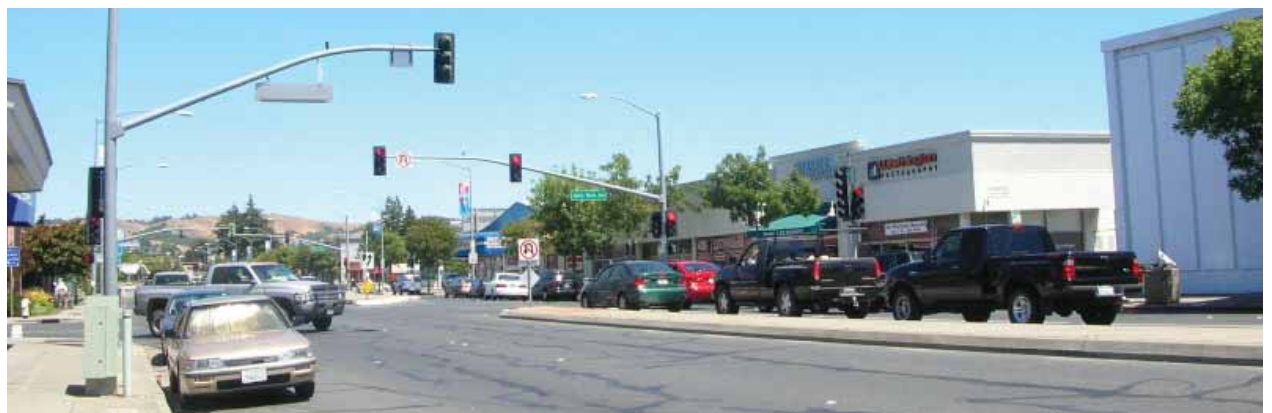
Photograph of Castro Valley Boulevard prior to streetscape improvements, shows the banal character of the street lacking a cohesive landscape treatment and basic public realm elements.
