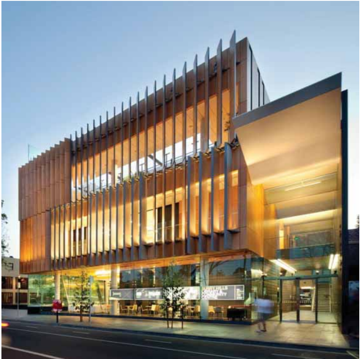
A well designed new academic building would serve as a beacon on Blackstone for the college and important catalyst.
