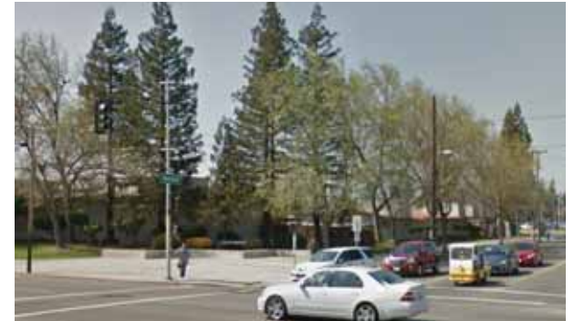
FCC maintenance facilities at Weldon and Blackstone Avenue do not create an active frontage at an important intersection.
