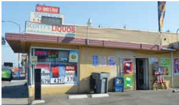
Single story liquor stores in cheaply constructed buildings are not a positive contributor to the street life.
