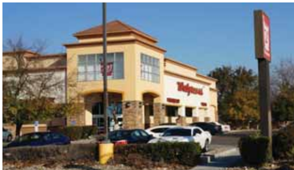
Even newer retail buildings do not have a street orientation and are surrounded by large surface parking.
