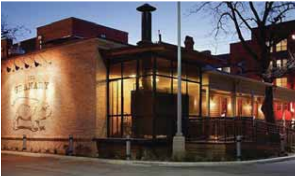
Existing buildings offer cost effective strategies for redevelopment.
