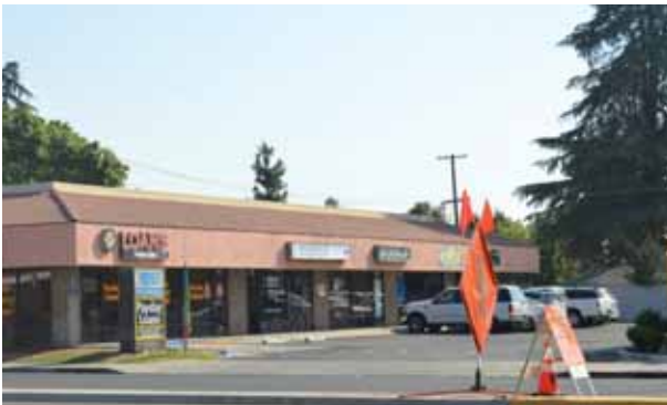
Most of the parcels on Blackstone Avenue within study area have small frontage, and are surrounded by large surface parking. Frequently occurring curbcuts create a conflict between pedestrians and vehicles.
