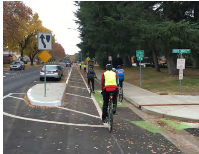
A clearly delineated buffer area provides sufficient space between the bicyclists' path of travel and the door zone of the adjacent parking lane.
