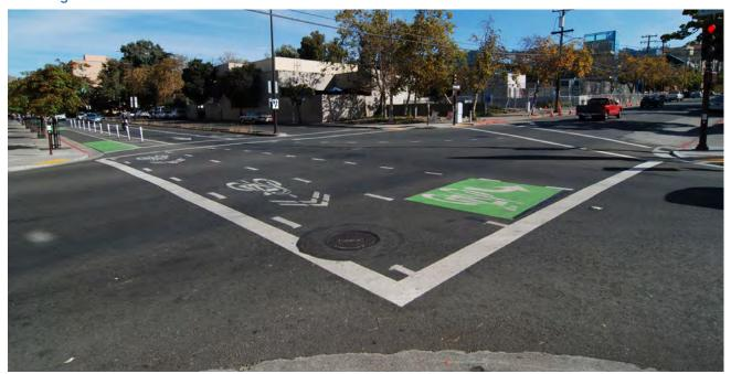
On separated bikeways, the two-stage turn box can be located in the protected buffer/parking area.
