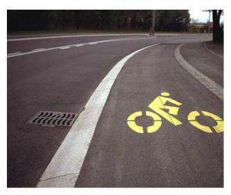
When adjacent to a travel lane, a one-way raised separated bikeway may be configured with a mountable curb. If used, the mountable curb should have a 4:1 slope edge. (NACTO Urban Bikeway Design Guide)
