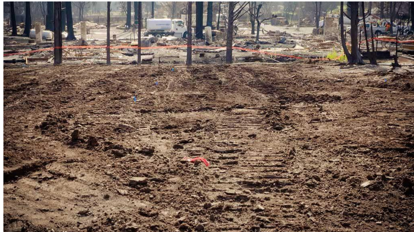
Figure 20: Post-Wildfire Debris Removal Northern California
