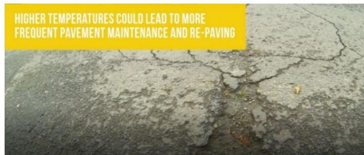
Figure 8: Impacts of Higher Temperature on Pavement
