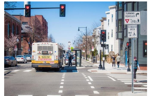
Figure 26: A concrete curb-separated bike lane (top); bike lane bending out to traverse behind transit boarding island (bottom).
