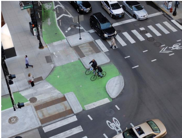
Figure 20: A separated bike lane in an intersection (left), and a graphic of a bicycle signal to protect bicyclists from right-turning traffic (right).
