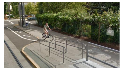
Figure 25: A separated bike lane transitioning to from on street to shared path/sidewalk behind a transit stop.
