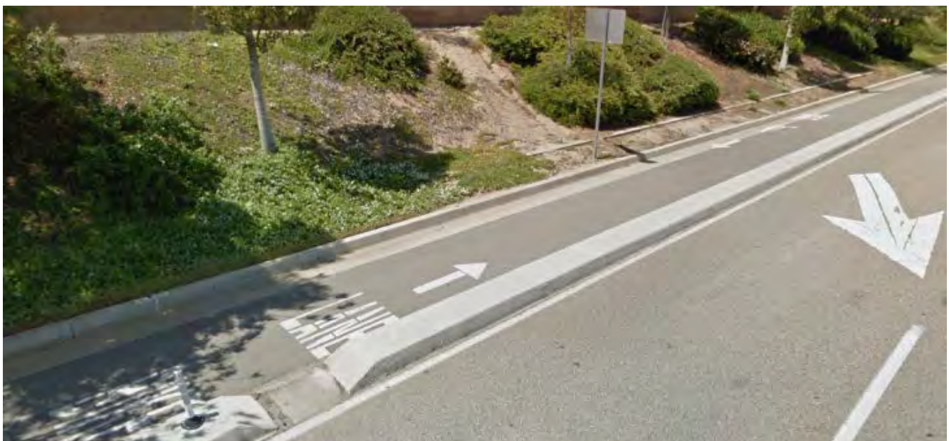
Two-way separated bikeway installation on Nighthawk Way, Source: Google
