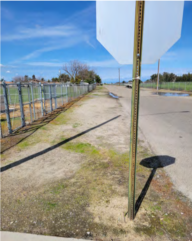
Figure 6: West side of Lily Ave facing north at elementary school.
