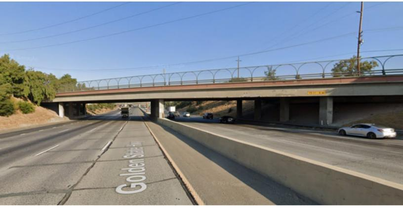
SR-99 underpasses can create hazardous conditions during flooding events, as they are below grade and at lower points in the urban drainage.
